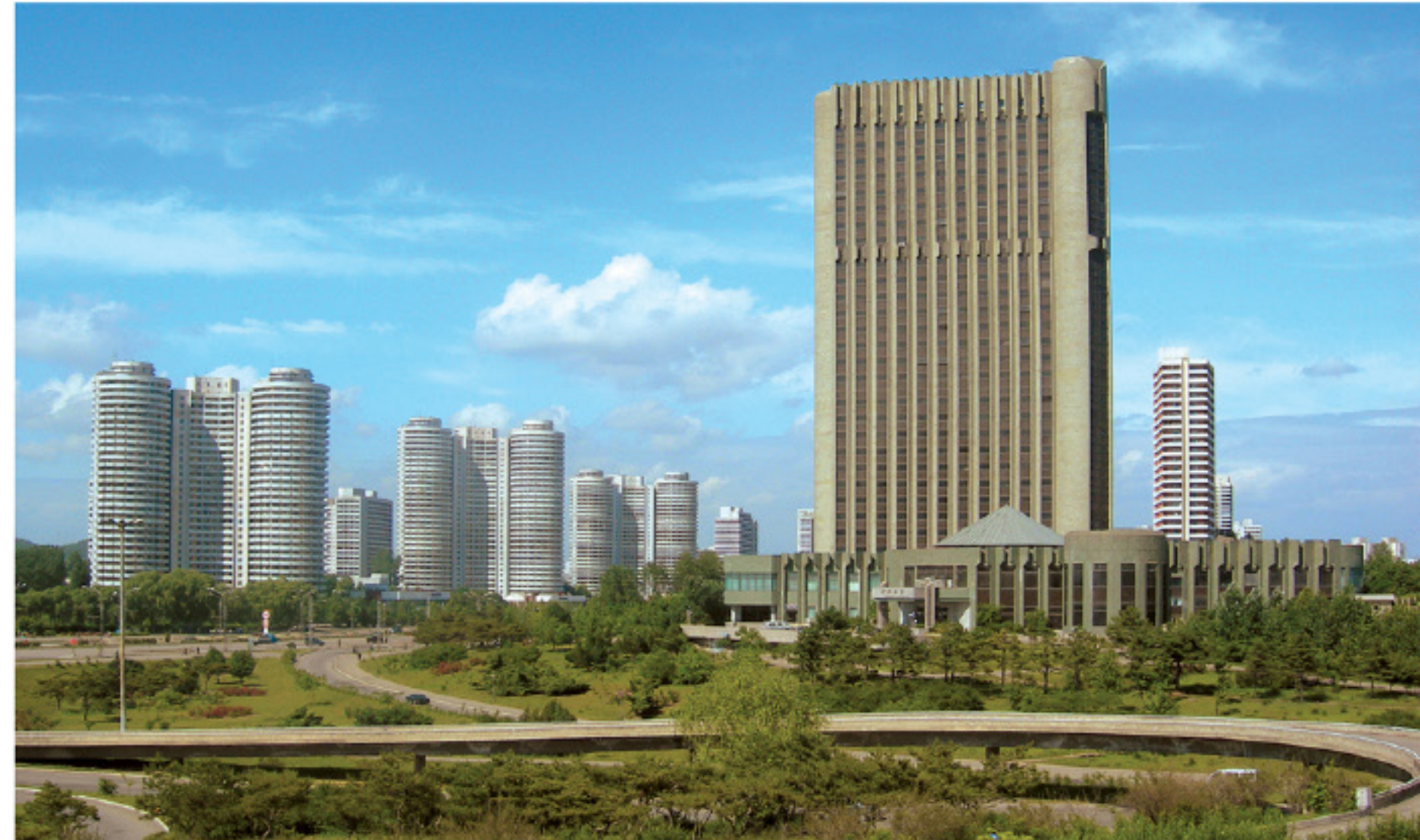
Partial view of Kwangbok Street
