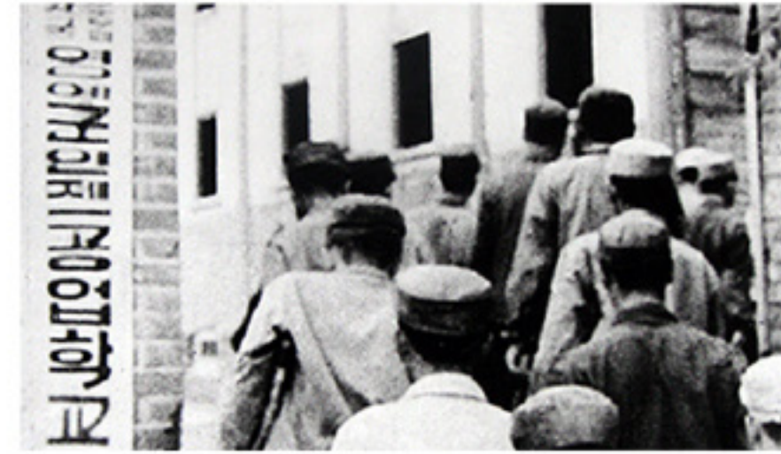
Students going to Technical School No. 1 for Honoured Disabled Soldiers set up in the wartime
